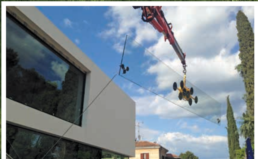
Schüco panorama ASS 77.PD.HI, AWS/ADS 75.SI, AWS/ADS 50.NI; Sliding shutters with TEAK by S.B.S. (wing ~3400 x 3300 mm); Low iron glass by Sedak ~600 m 2 with AGC coating ipasol ultraselect 62/29 and glass balustrades XXL glass dimension: 8885 x 3045 mm, 7530 x 3045 mm, 6640 x 3045 mm, 5860 x 3045 mm, 5425 x 3045 mm, 8570 x 1155 mm, 7515 x 1140 mm ...
