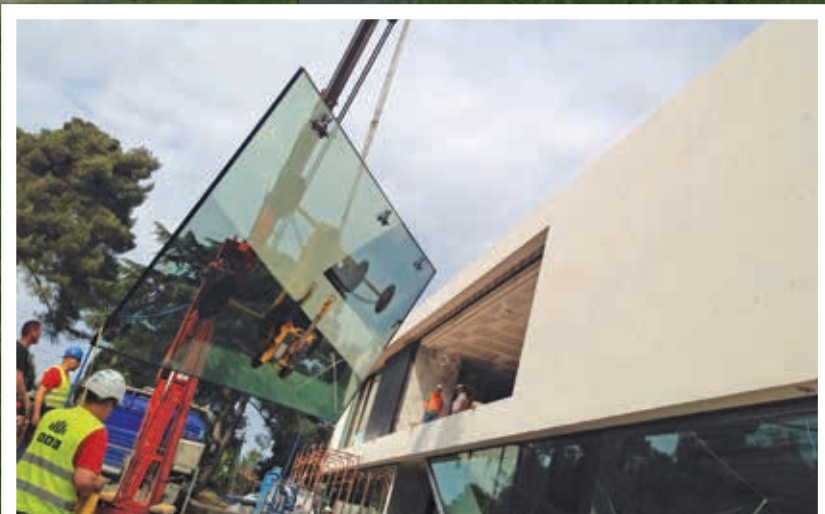
Schüco panorama ASS 77.PD.HI, AWS/ADS 75.SI, AWS/ADS 50.NI; Sliding shutters with TEAK by S.B.S. (wing ~3400 x 3300 mm); Low iron glass by Sedak ~600 m 2 with AGC coating ipasol ultraselect 62/29 and glass balustrades XXL glass dimension: 8885 x 3045 mm, 7530 x 3045 mm, 6640 x 3045 mm, 5860 x 3045 mm, 5425 x 3045 mm, 8570 x 1155 mm, 7515 x 1140 mm ...
